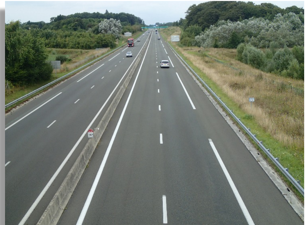
Autoroute A16 Forest-Montiers
